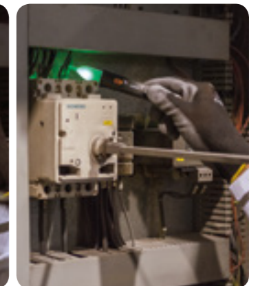
Step3 - If the green LED turns on with steady light, phase sequence is correct . If, however, the red LED flashes, phase sequence is incorrect .
