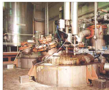
Batching Processes Reactors and Process Vessels
